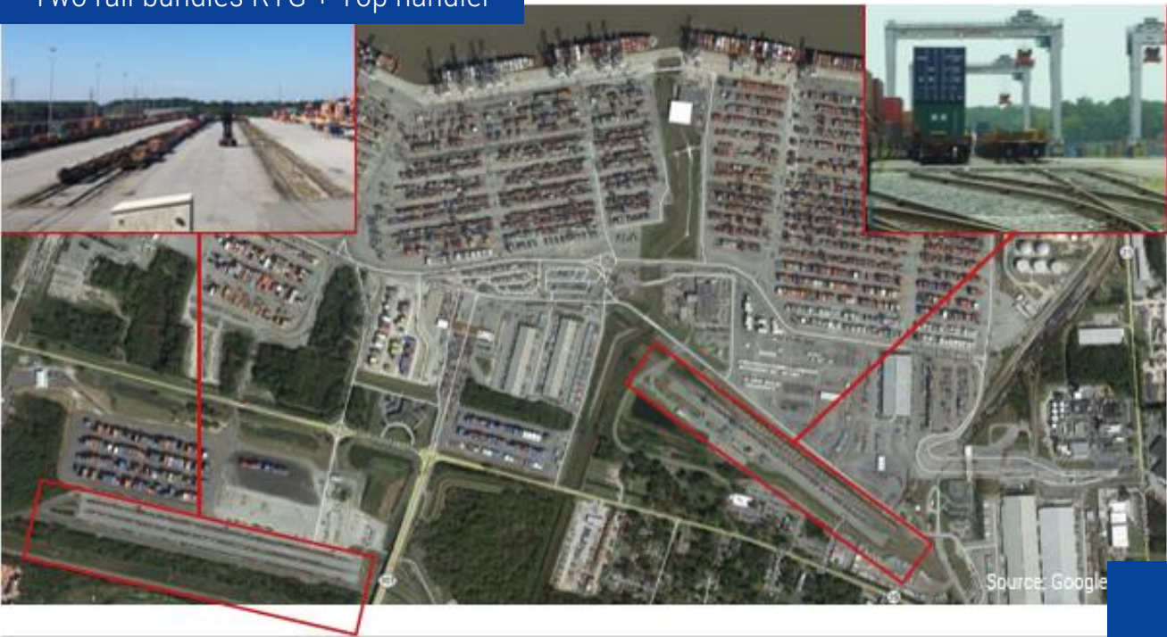
Two rail bundles RTG + Top handler
